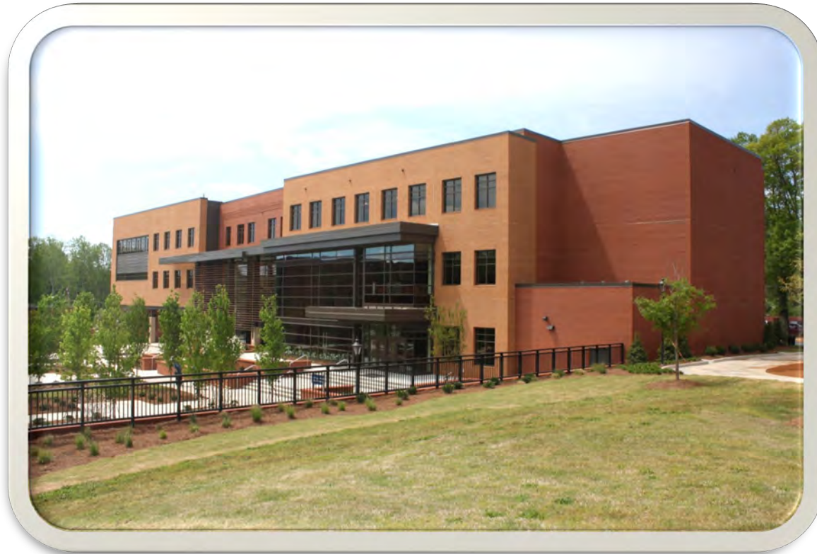
Nursing and Allied Health Sciences Building - April 2011
